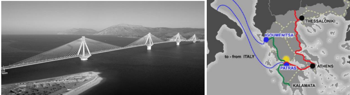
Figure 1 - The Rion – Antirion Bridge and the national road transport network its location (source: www.iabse.gr accessed on 16/07/2009 and Pilassi du Rausas, 2006)
